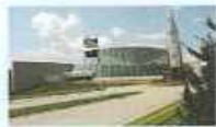
The glass atrium of 525 glass panels on the Strategic Air & Space Museum was built around the Lockheed SR-71 Blackbird.
