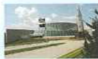
The glass atrium of 525 glass panels on the Strategic Air & Space Museum was built around the Lockheed SR-71 Blackbird.
